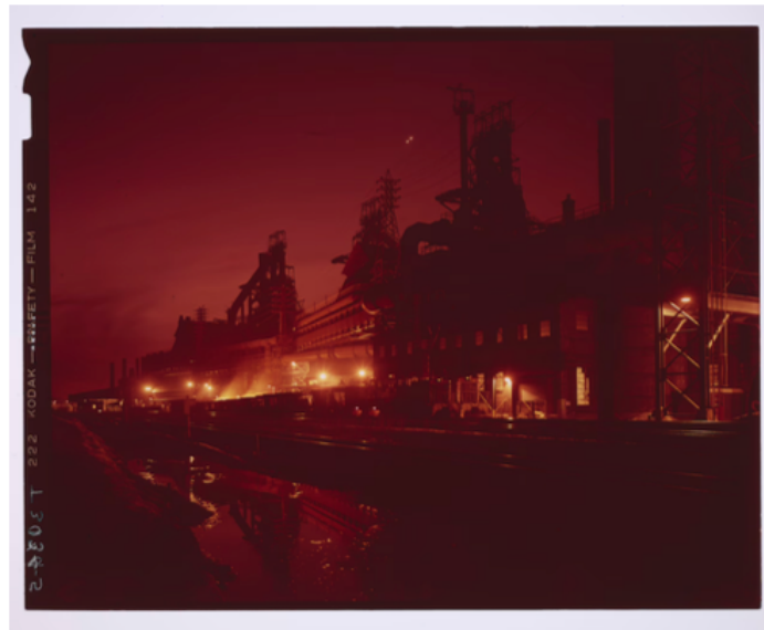
Bethlehem Steel Plant, 1964, Digitized by the National Museum of Industrial History, Bethlehem, PA.
